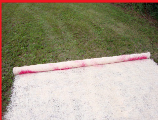
Locate red line near the end of the ECB.
