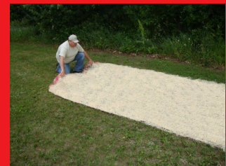
Properly position unrolled ECB for installation
